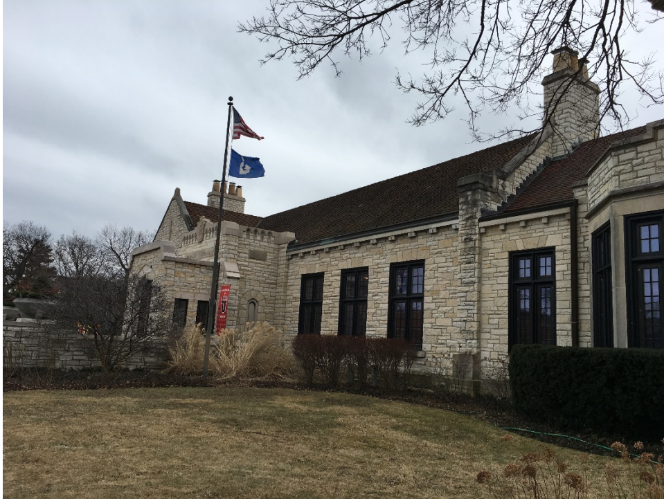
Existing Highland Park Library building.
