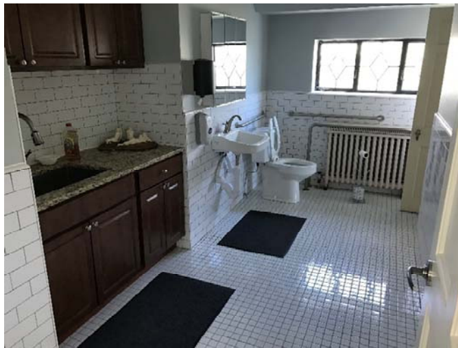
The facility's only accessible restroom is located on the second floor and is within a shared space with a sink and storage for the adjacent art studio.
