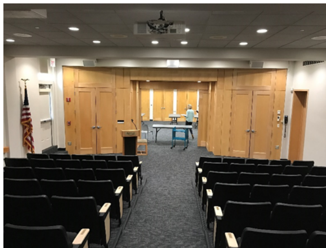
Adjacent auditorium with lower level meeting room beyond; sound transmission at door between auditorium and meeting room makes it impossible to hold programs in both spaces simultaneously.
